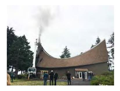
Demolition crews disassembled the roof structure. They preserved the original hardware and structural plates to be refinished and reused in preparation for the new, custom glulam beams.
